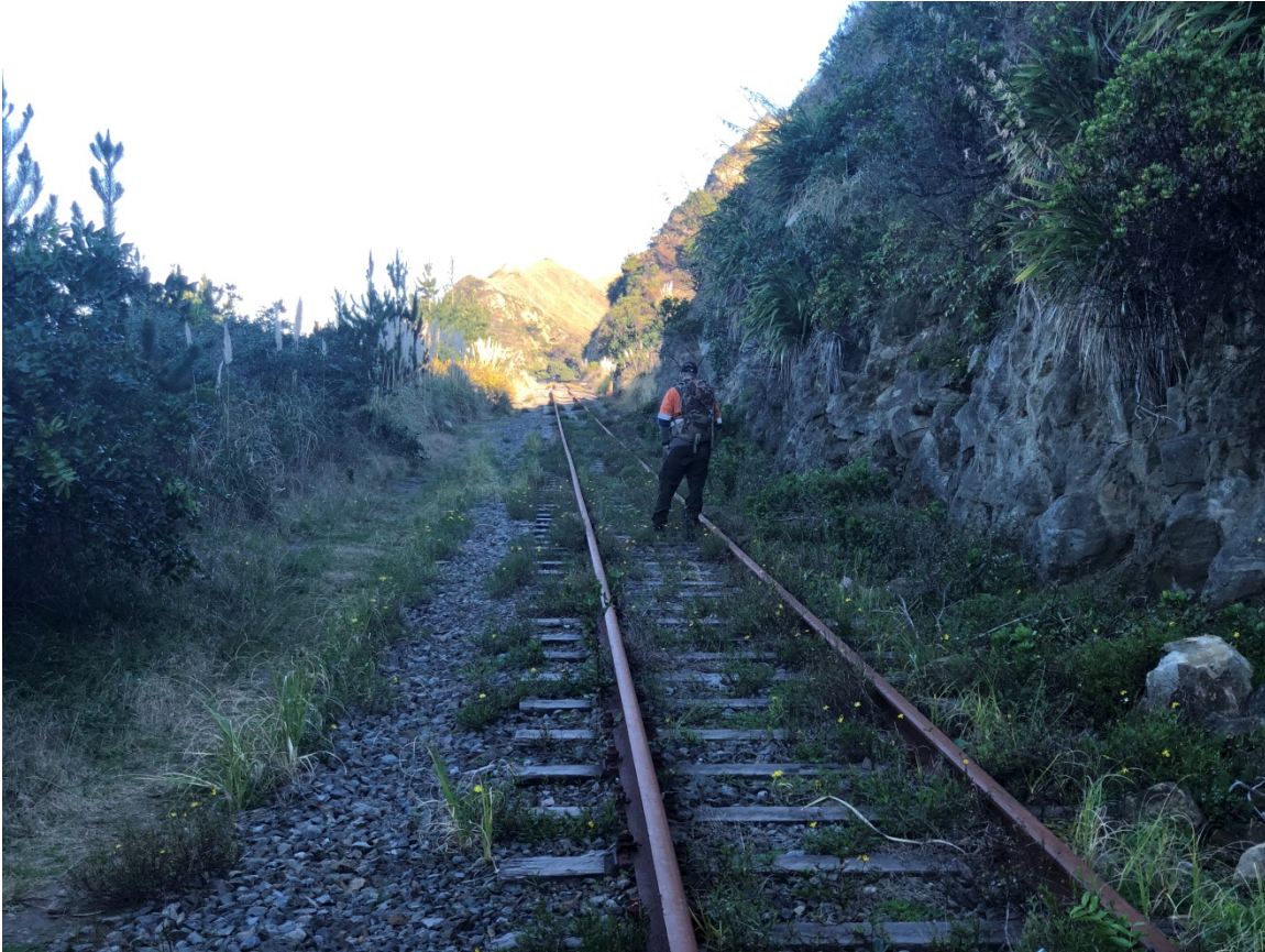
View of track looking south to bridge 261 – note relatively limited drop rock in side swales.
