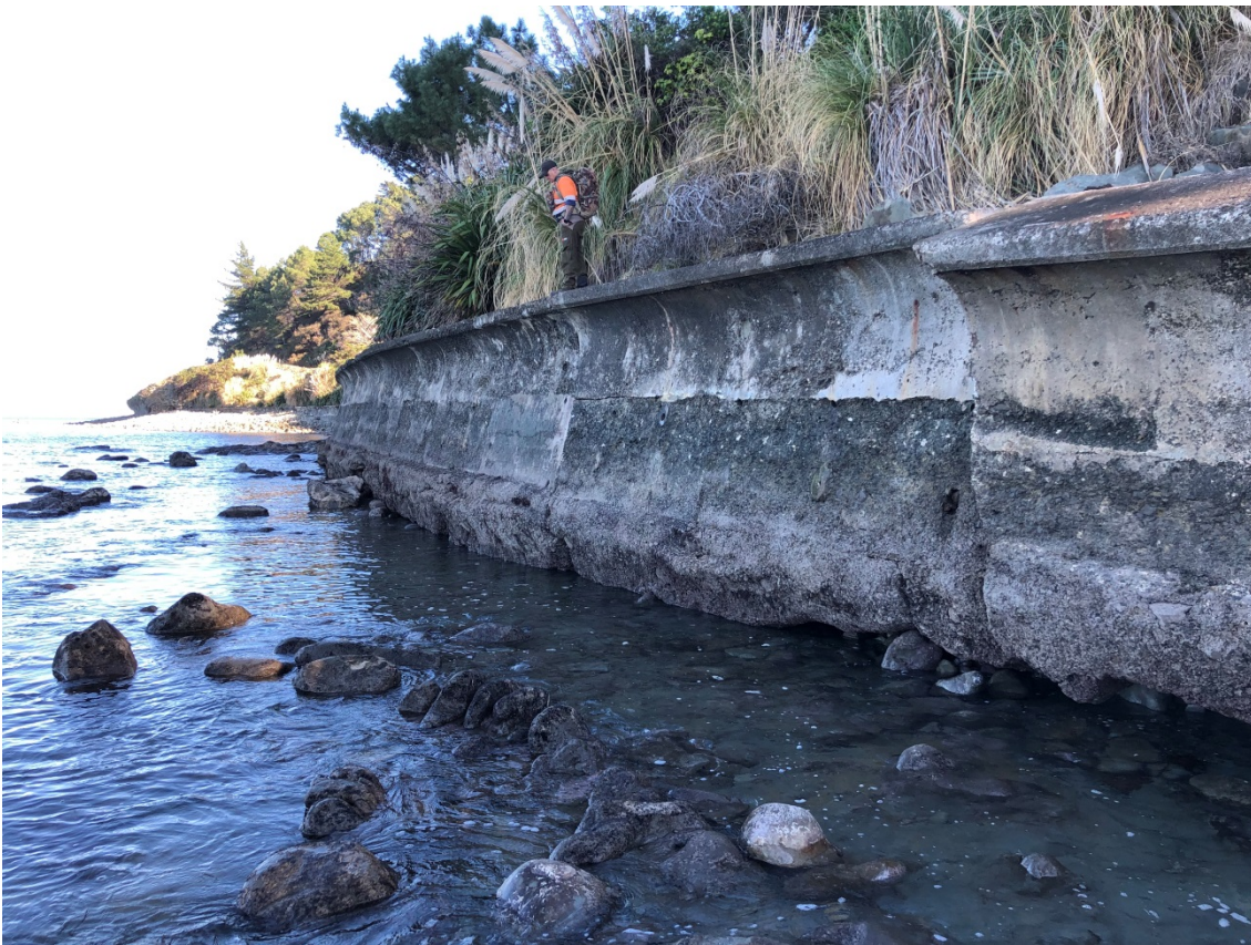
Typical photos of toe erosion and wall over topping erosion
