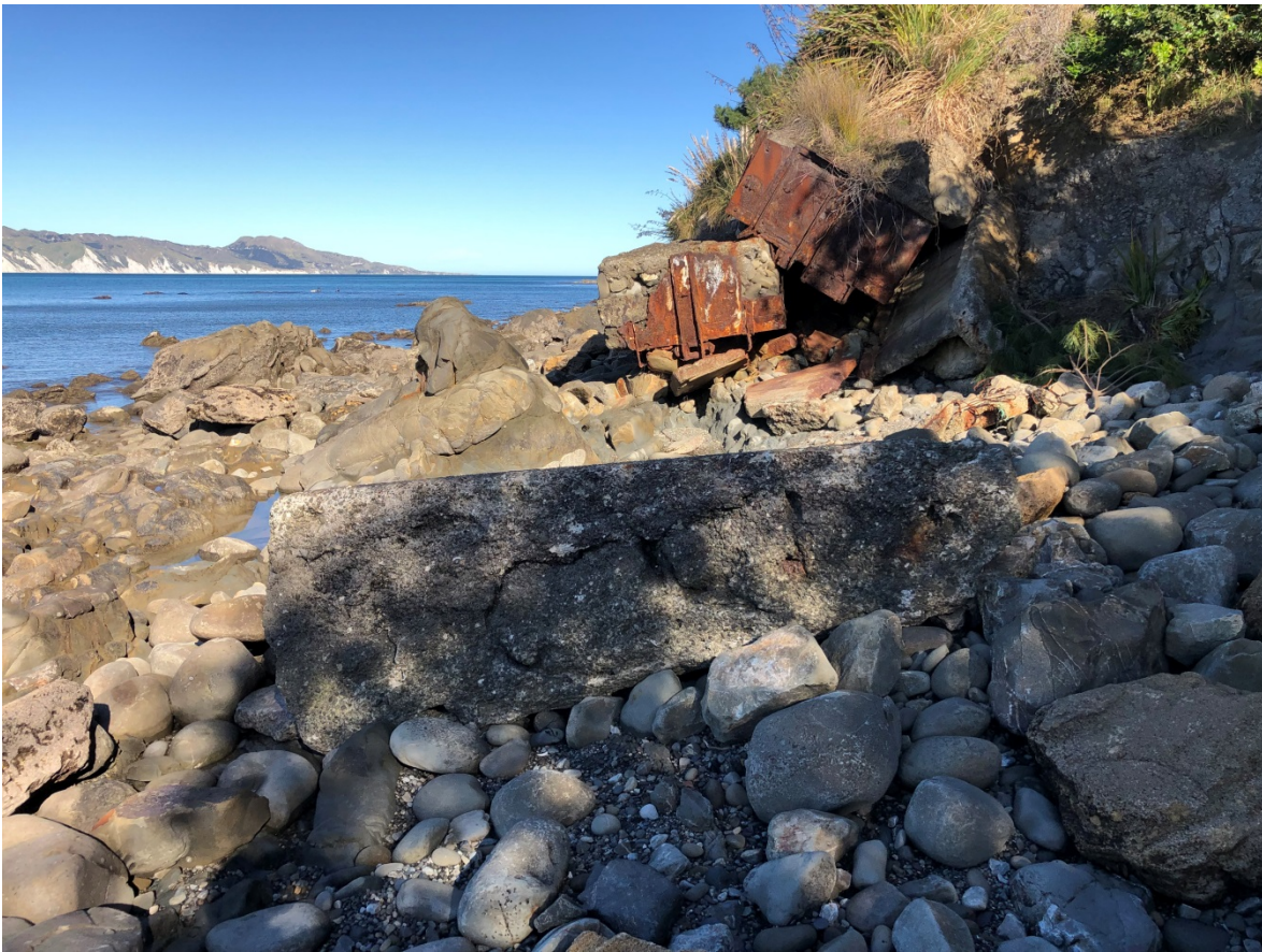
View looking south into railway wagon erosion protection
