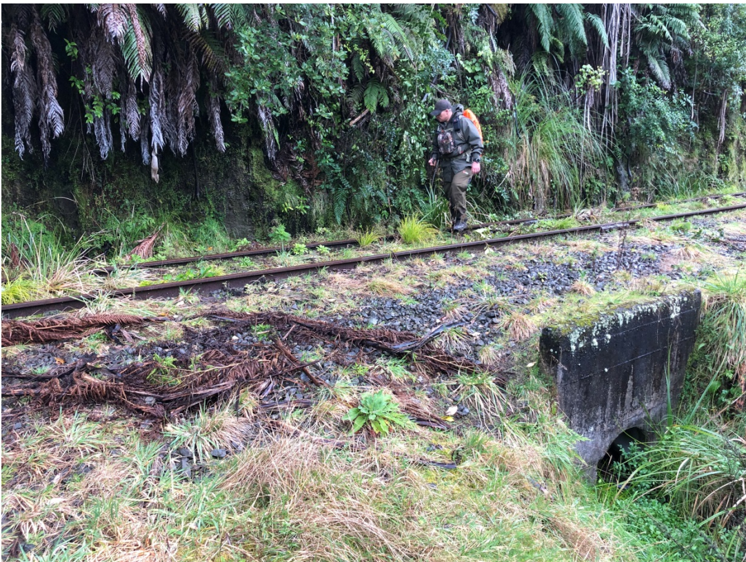
Typical culvert and swale photos in area of interest – note heavily blocked swales, blocked culvert inlets and outlets, over grown vegetation.
