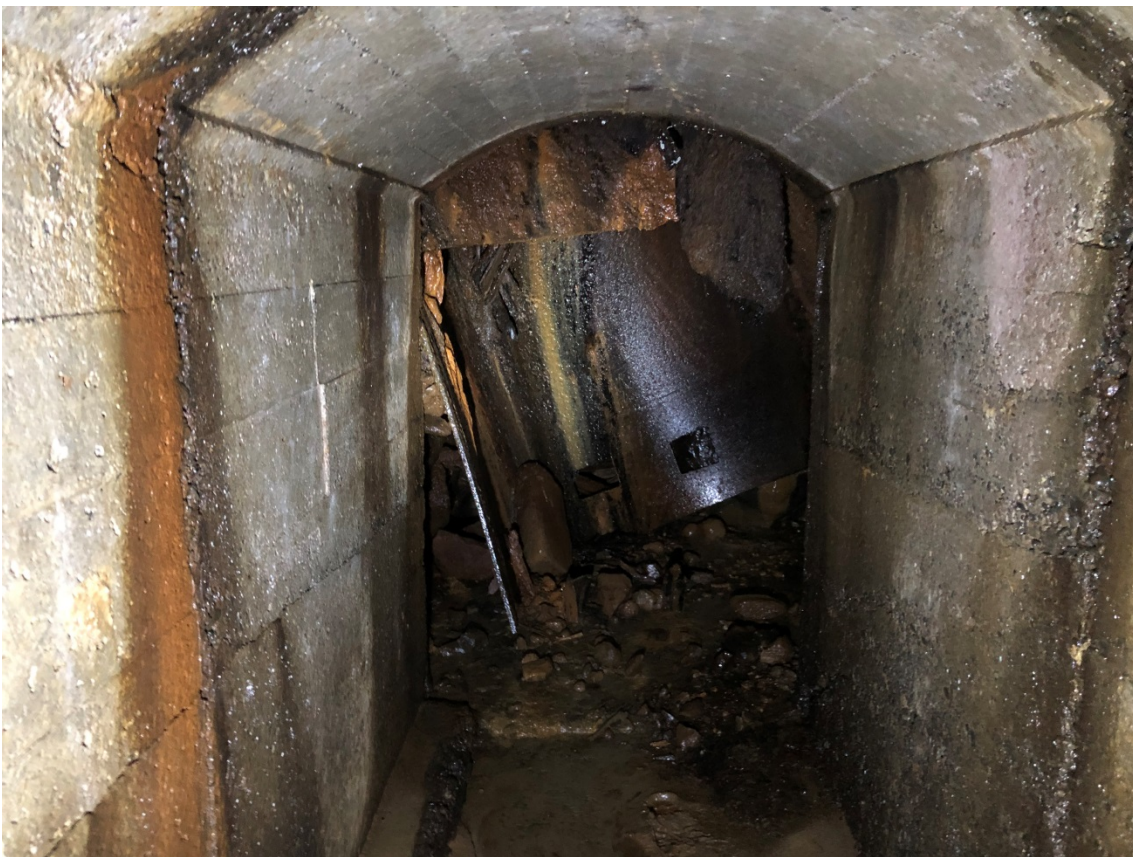
1.22 wide by 1.8m high arch culvert, 30m long @ upstream end. Note blocked inlet
