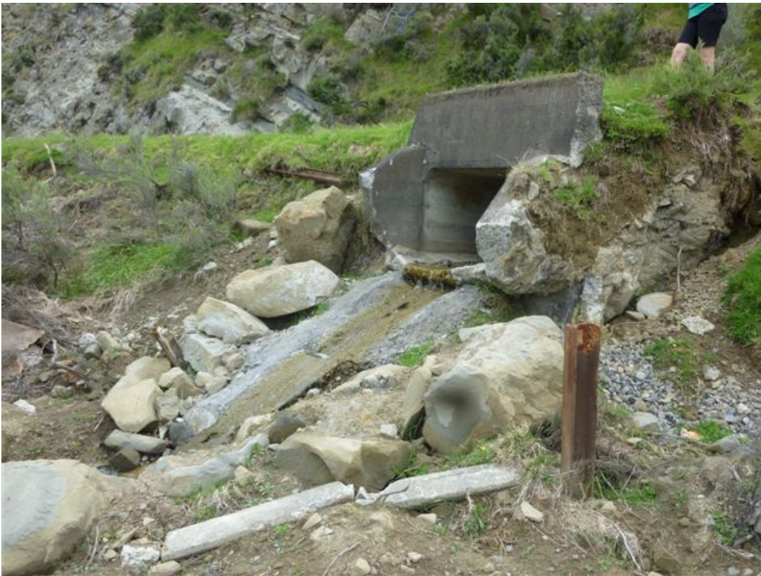
Outlet culvert@ 355.516km – 2013 photo above, 2019 photo below. Note slope movement / head scarp and ground pulling away from under culvert edge. Nominal 400mm downwards movement over 6 years due to water getting into slope from culvert discharge
