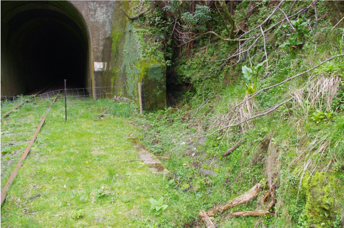
2013 Photographs – blocked swale drainage and culvert inlet (assumed 355.420km location)
