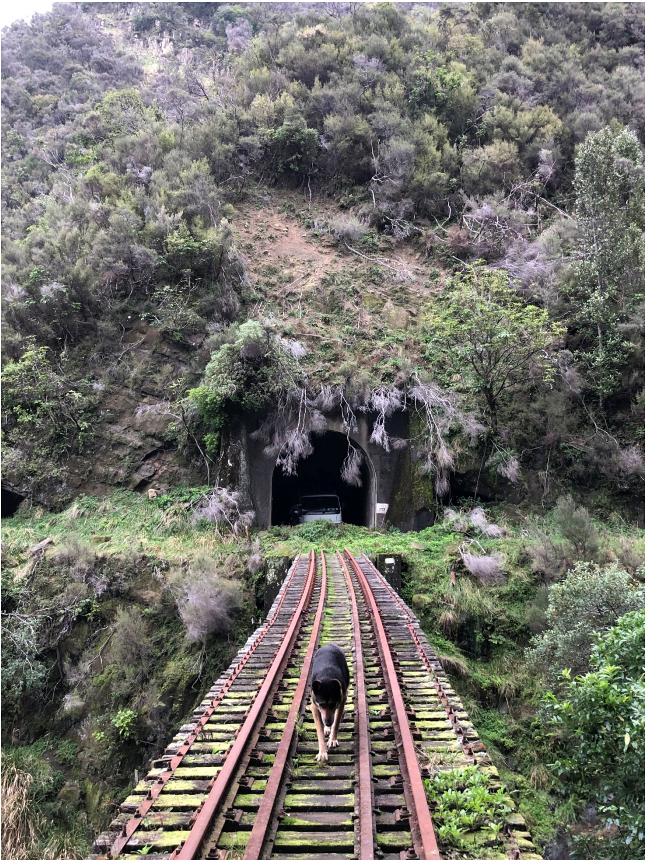
View looking into Tunnel 19 northern portal – note minor slip above portal entrance with debris on track. Bridge 268A in foreground.
