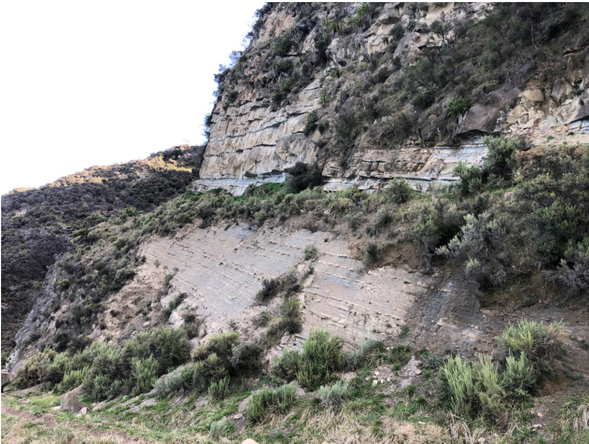
Views of rock face north of dropout 3 – note catch bench in above photo (requires clearance)-.
