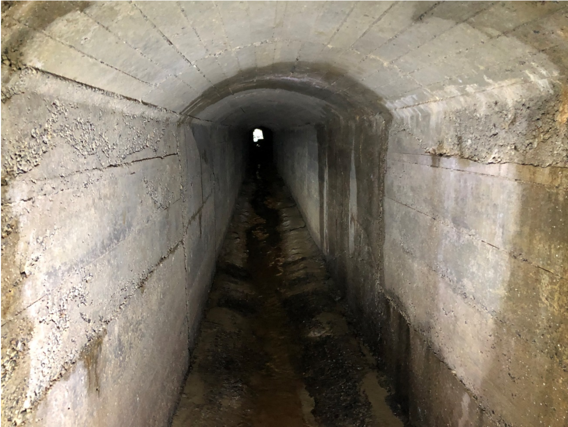
1.22 wide by 1.8m high arch culvert, 30m long @ upstream end. Note blocked inlet
