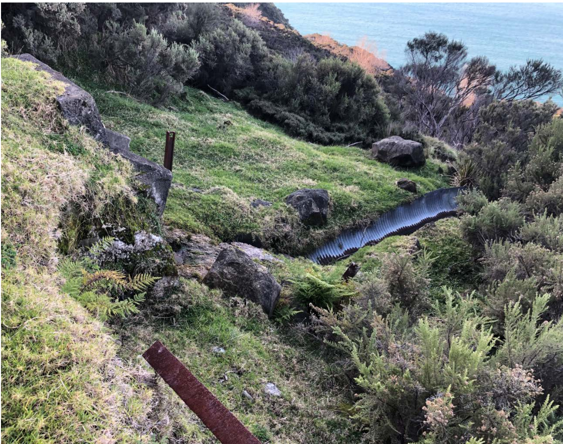
Existing flume details – require upgrading and replacement
