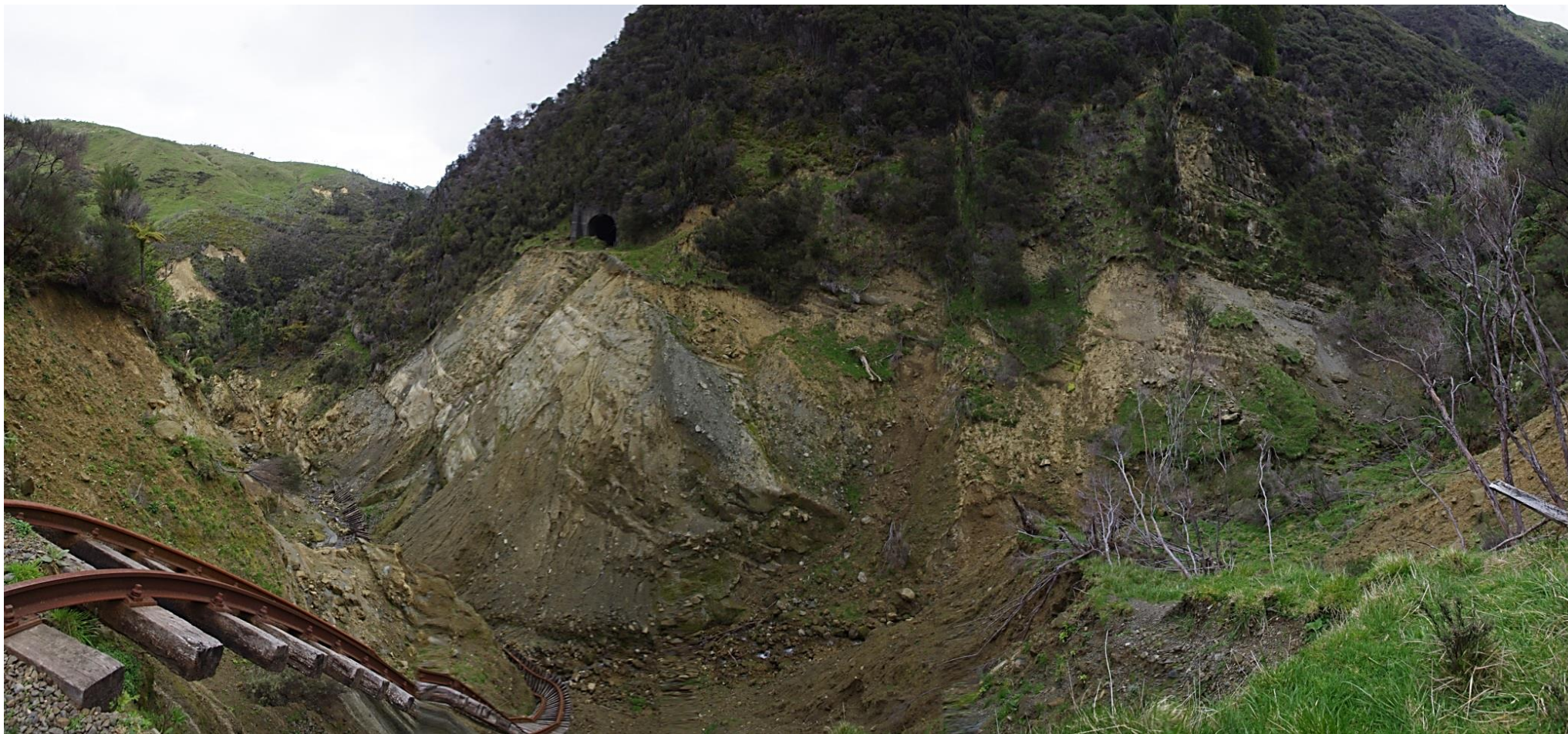
2013 view looking south. Note remnant tunnel spoil in base of gully along base of southern facing – this is mostly eroded away in 2019 photos
