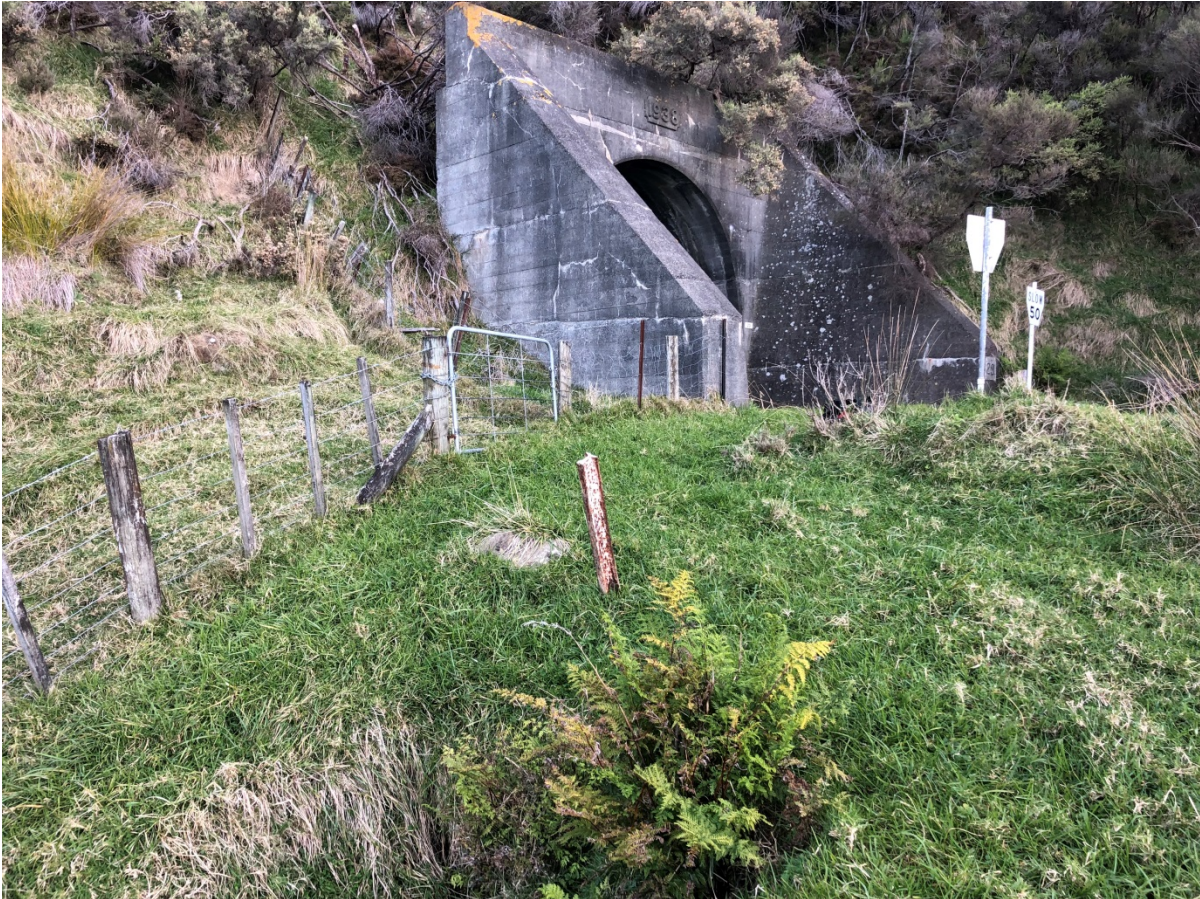
Tunnel 23 drainage outlet in picture foreground – requires cleanout.
