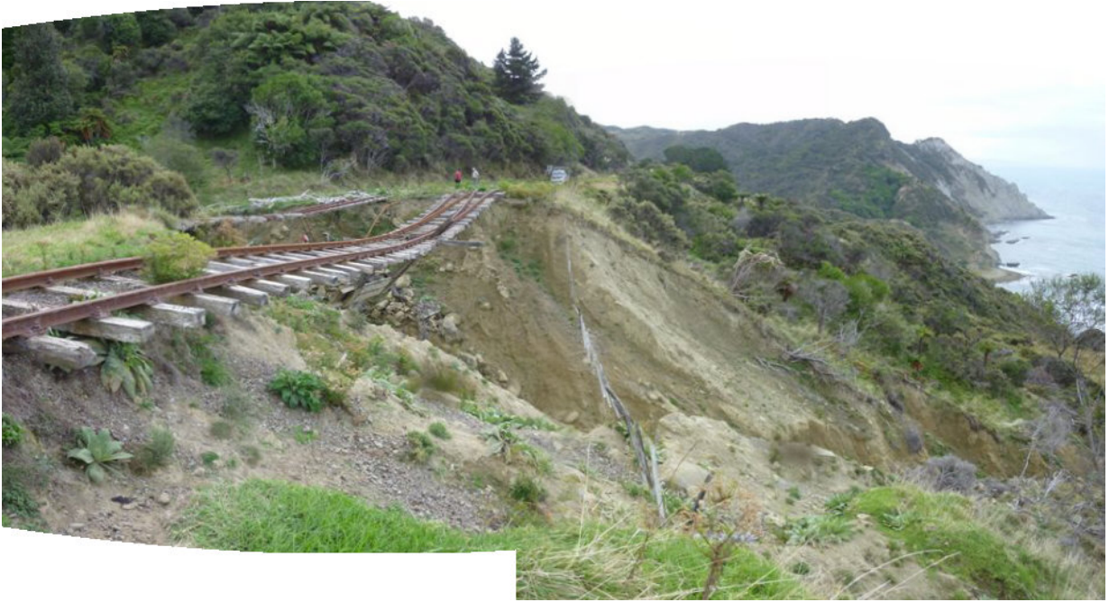
Stitched photo view looking north - note extensive spoil depths on far facing, no intact rockmass visible.
