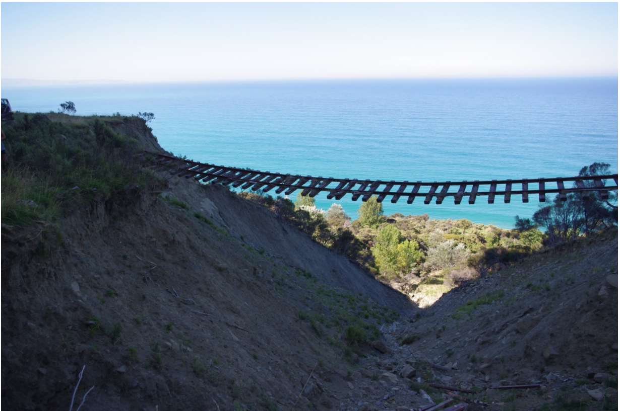
Stitched photo view looking north - note extensive spoil depths on far facing, no intact rockmass visible.
