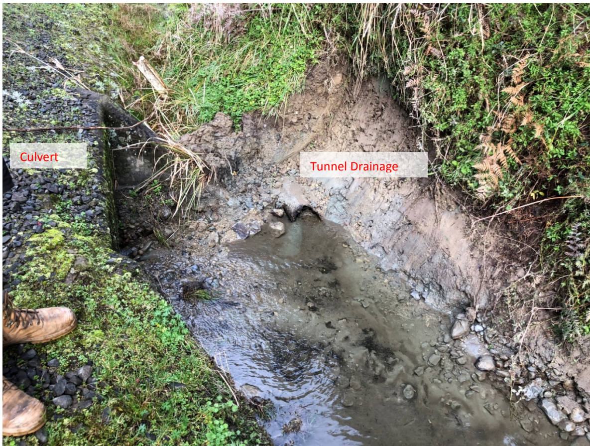
Uncovered tunnel drainage on western side of formation, plus flow through culvert under track.
