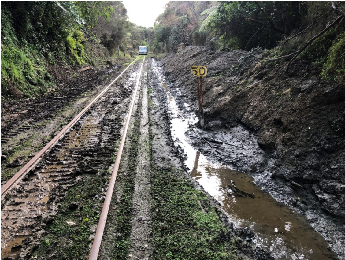
Temporary drainage works undertaken in week of 15 July 2019 – open up tunnel drainage, stockpile spoil against stream to confine sediment to channel and stop water flooding over track. Note significant groundwater drainage flowing out of exposed ballast.
