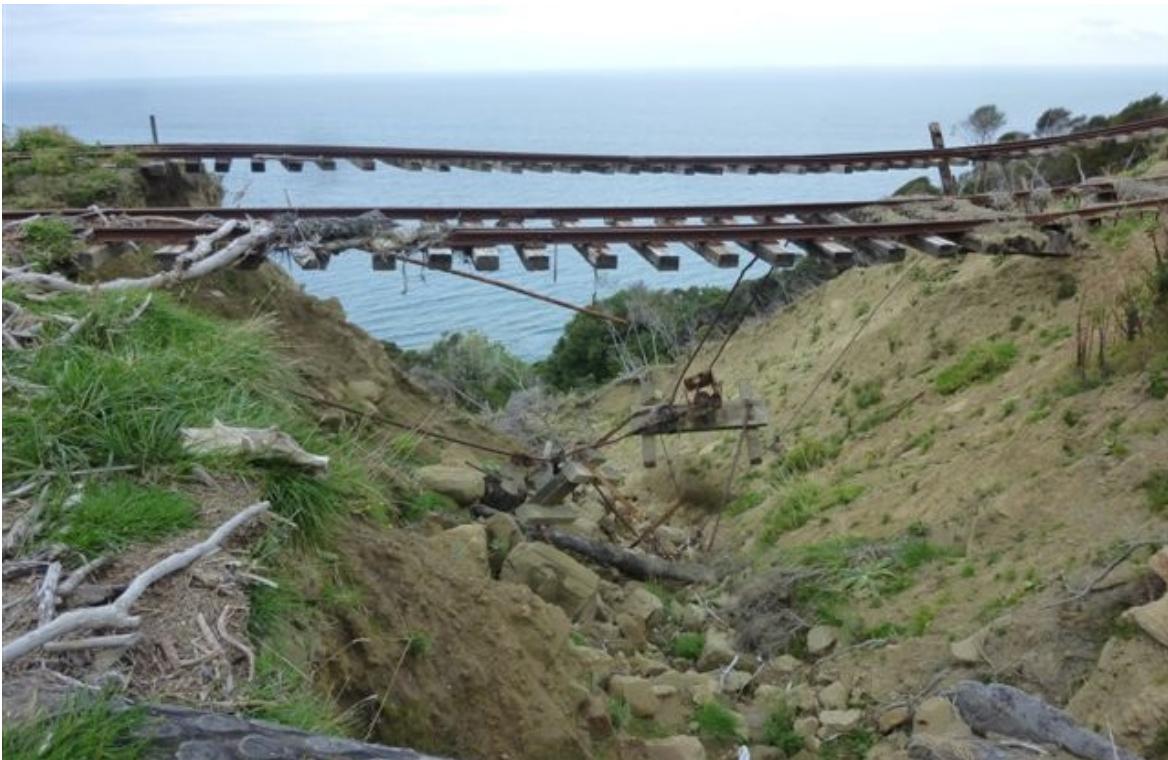
2013 photographs – extent of washout and track formation damage. Base of dropout is still in spoil - no hard rock visible in photographs or during inspections.
