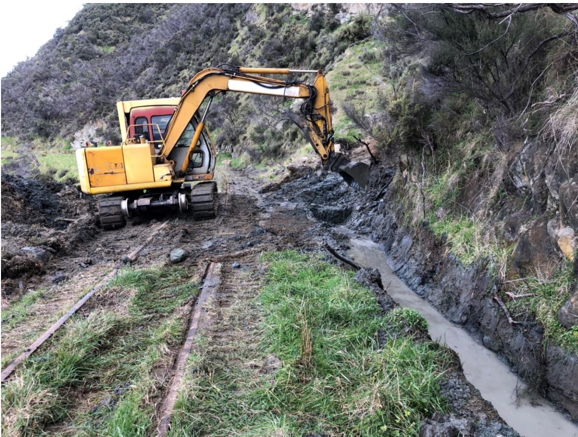
Swale clearance works July 2019 to prevent water flooding across track and destabilising slope on outside edge of track formation.
