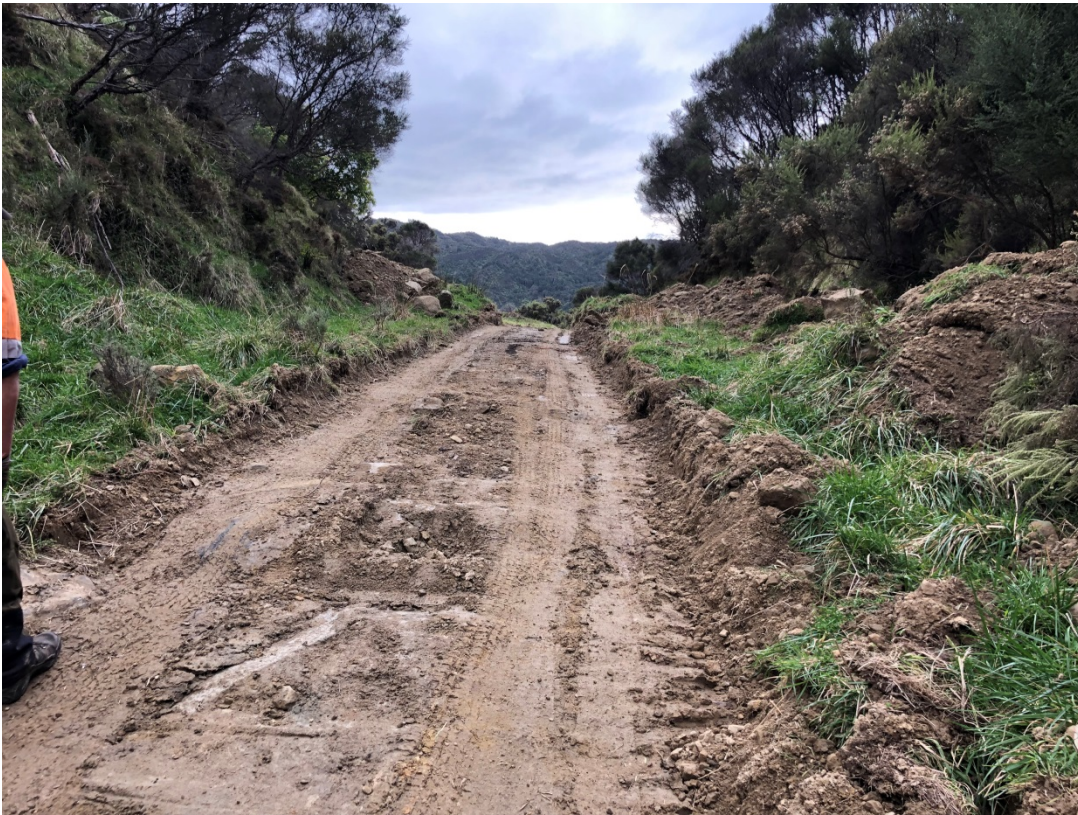
2019 Photos showing temporary access track across top of spoil (note large spoil volume)
