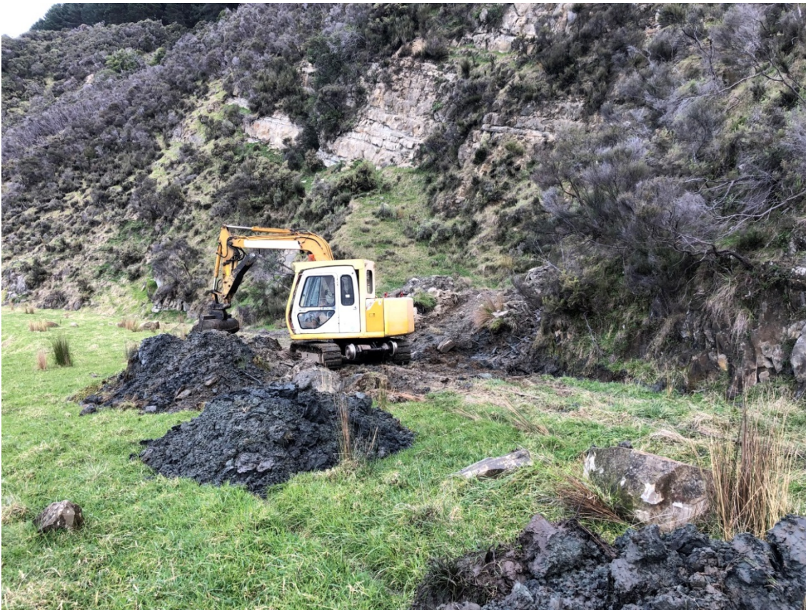
Swale clearance works July 2019 to prevent water flooding across track and destabilising slope on outside edge of track formation.
