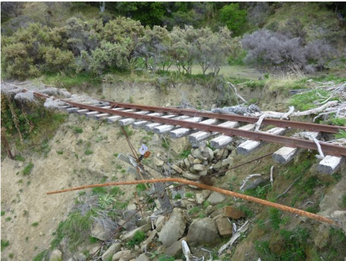
2013 photographs – extent of washout and track formation damage. Base of dropout is still in spoil - no hard rock visible in photographs or during inspections.
