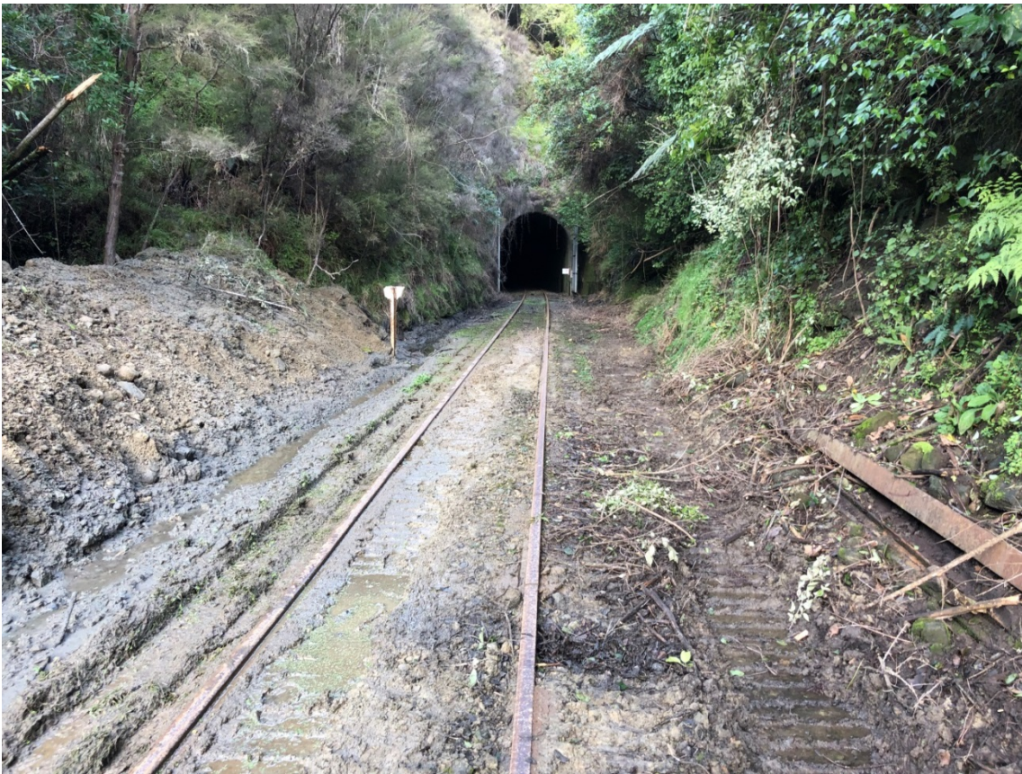
Temporary drainage works undertaken in week of 15 July 2019 – open up tunnel drainage, stockpile spoil against stream to confine sediment to channel and stop water flooding over track. Note significant groundwater drainage flowing out of exposed ballast.
