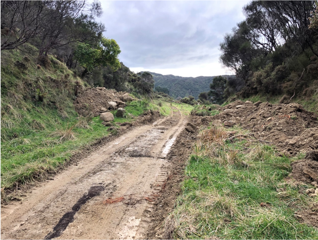
2019 Photos showing temporary access track across top of spoil (note large spoil volume)
