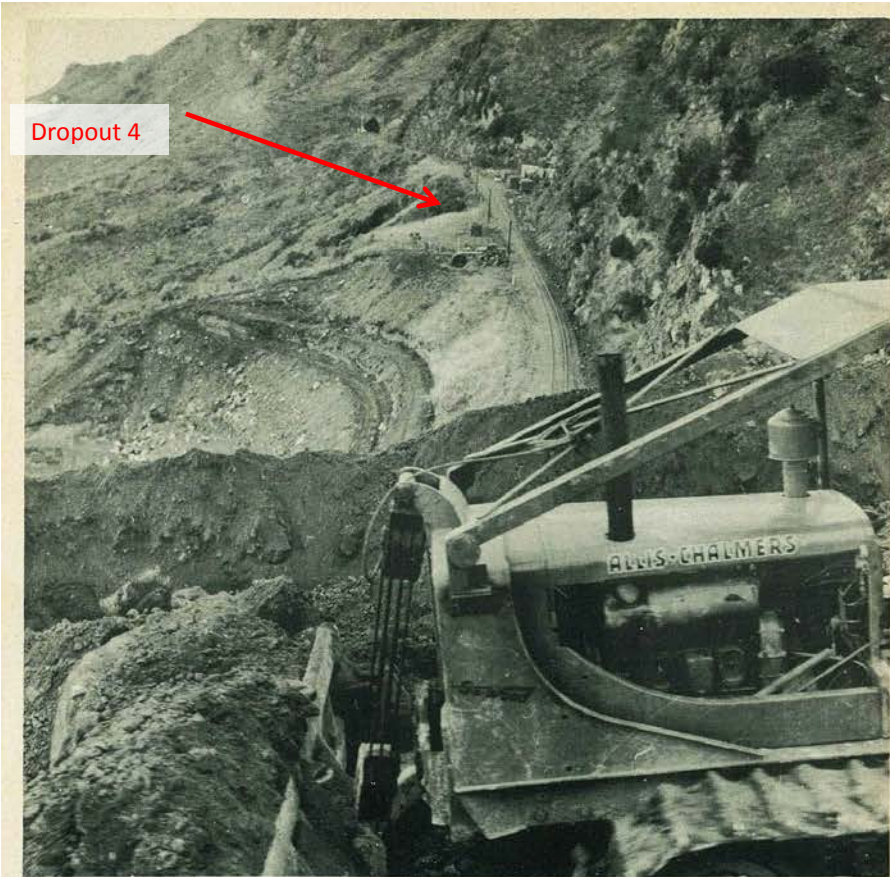
Above: View from shelf looking over bulldozer at work shows line snaking towards longer tunnel to south of job and workers' camp to right of line. Bulldozer is right over tunnel. Hill-side below line has been terraced to take embankment where new line will be laid. Left: Doug Herbison, of Whararata, on whose property work is being done, and who drove "Photo News" cameraman over rugged hills to job, chats with one of the bulldozer drivers. Contractors for job are Brooks and Tollison Ltd., Napier. They have only three months in which to complete the work.
